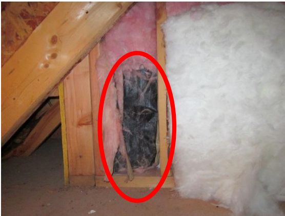
Damaged insulation and chewed wiring.
