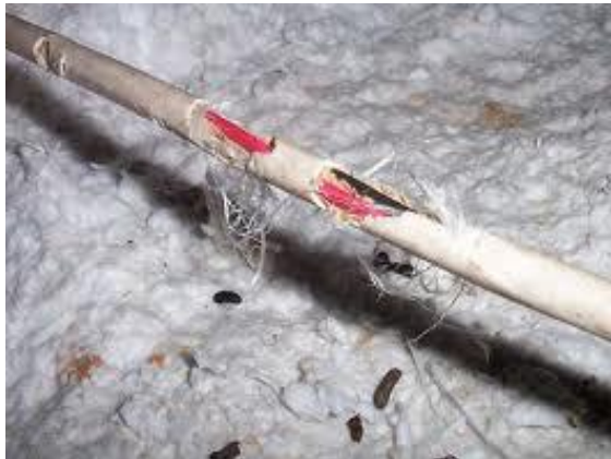
Damaged insulation and chewed wiring.
